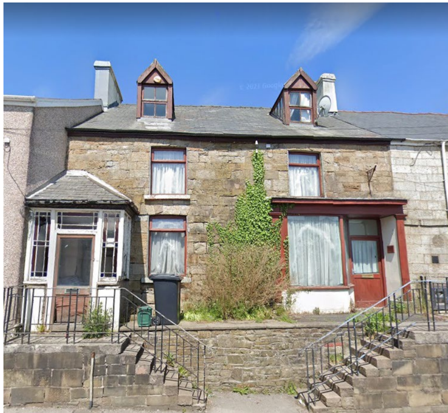
Fig. 1.1 Existing Property at 74 A King Street
